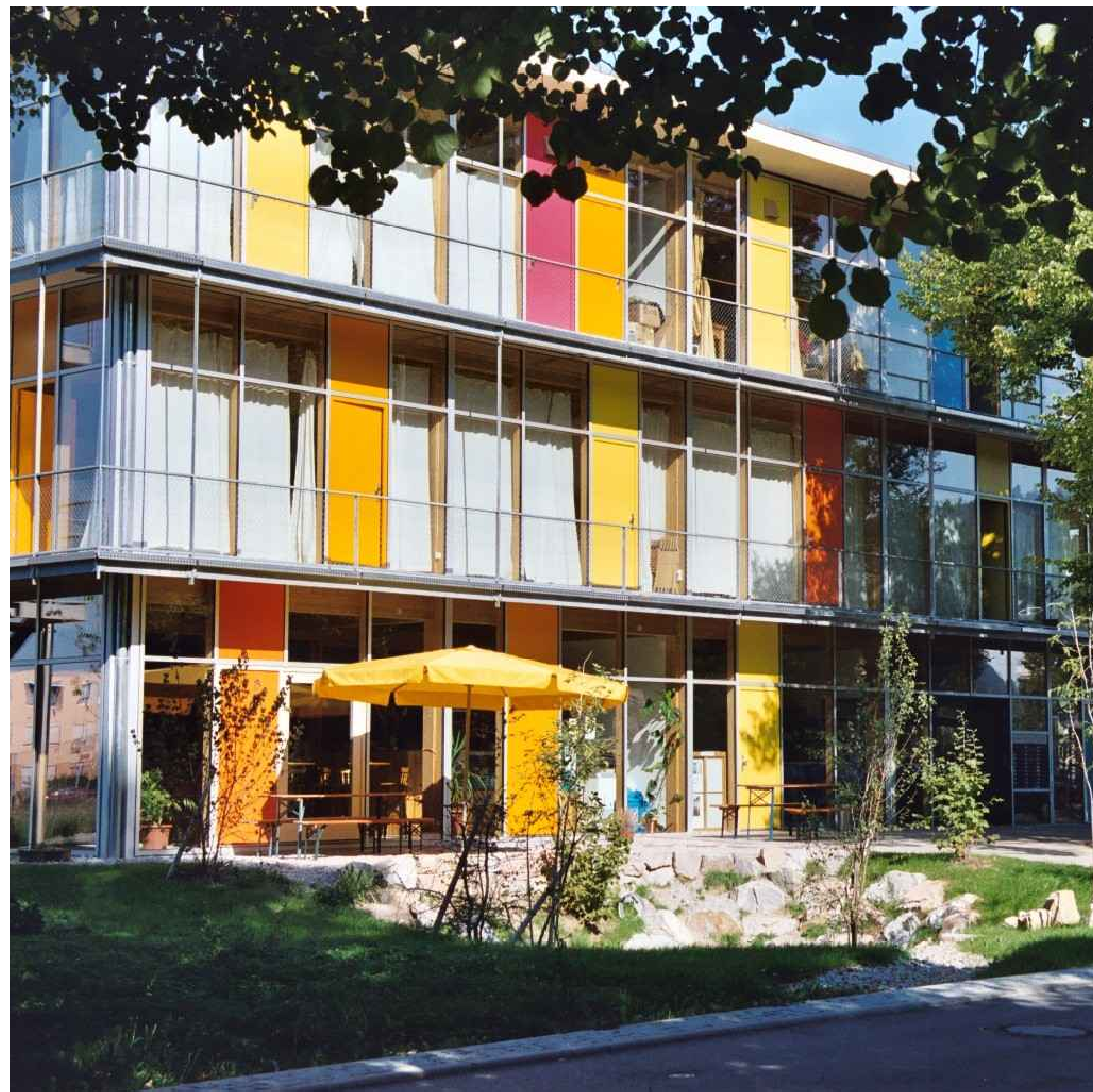
Marie-Curie-Straße / Gewerbeobjekt einer privaten Bauherrngemeinschaft - Commercial property constructed by a group of building-owners
