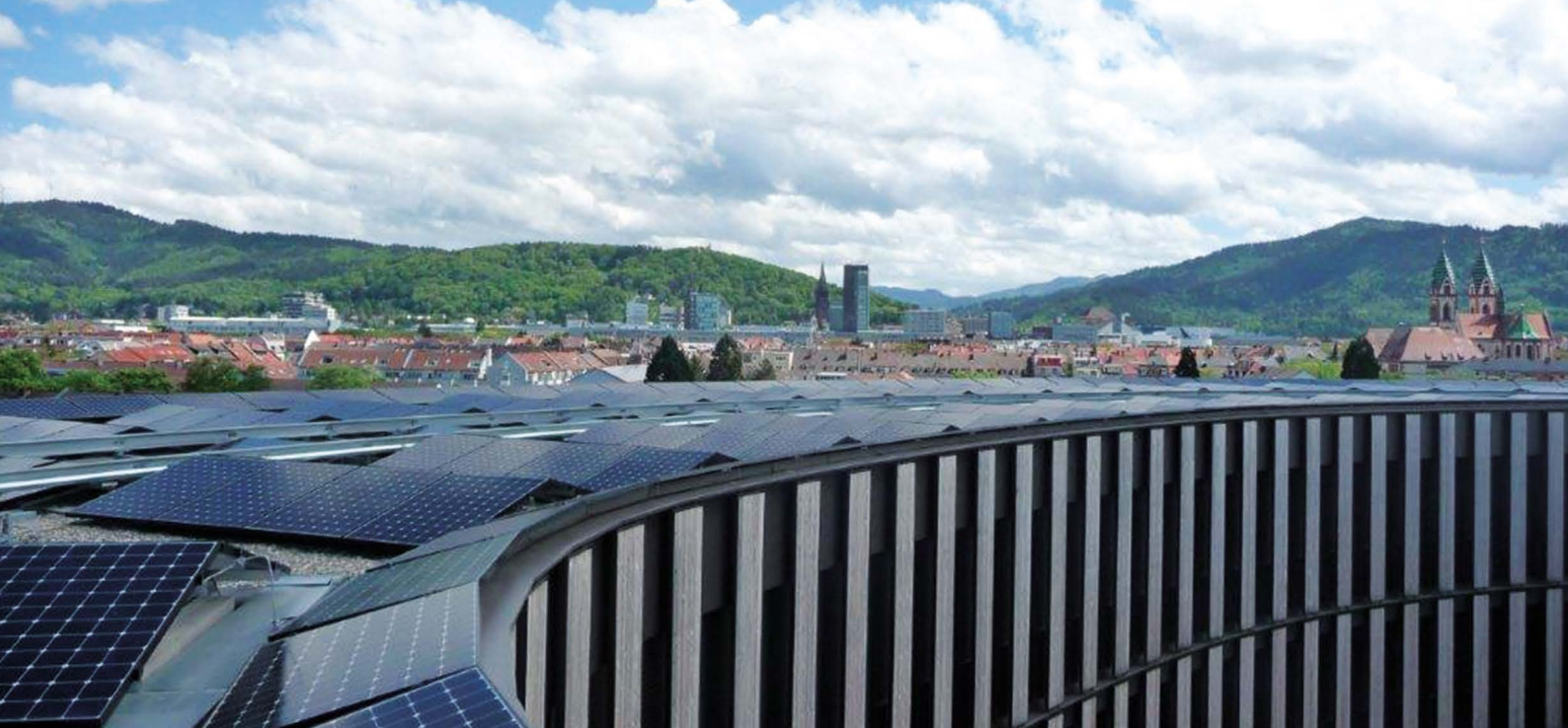
Solar system on the roof of the City Hall in Stühlinger
