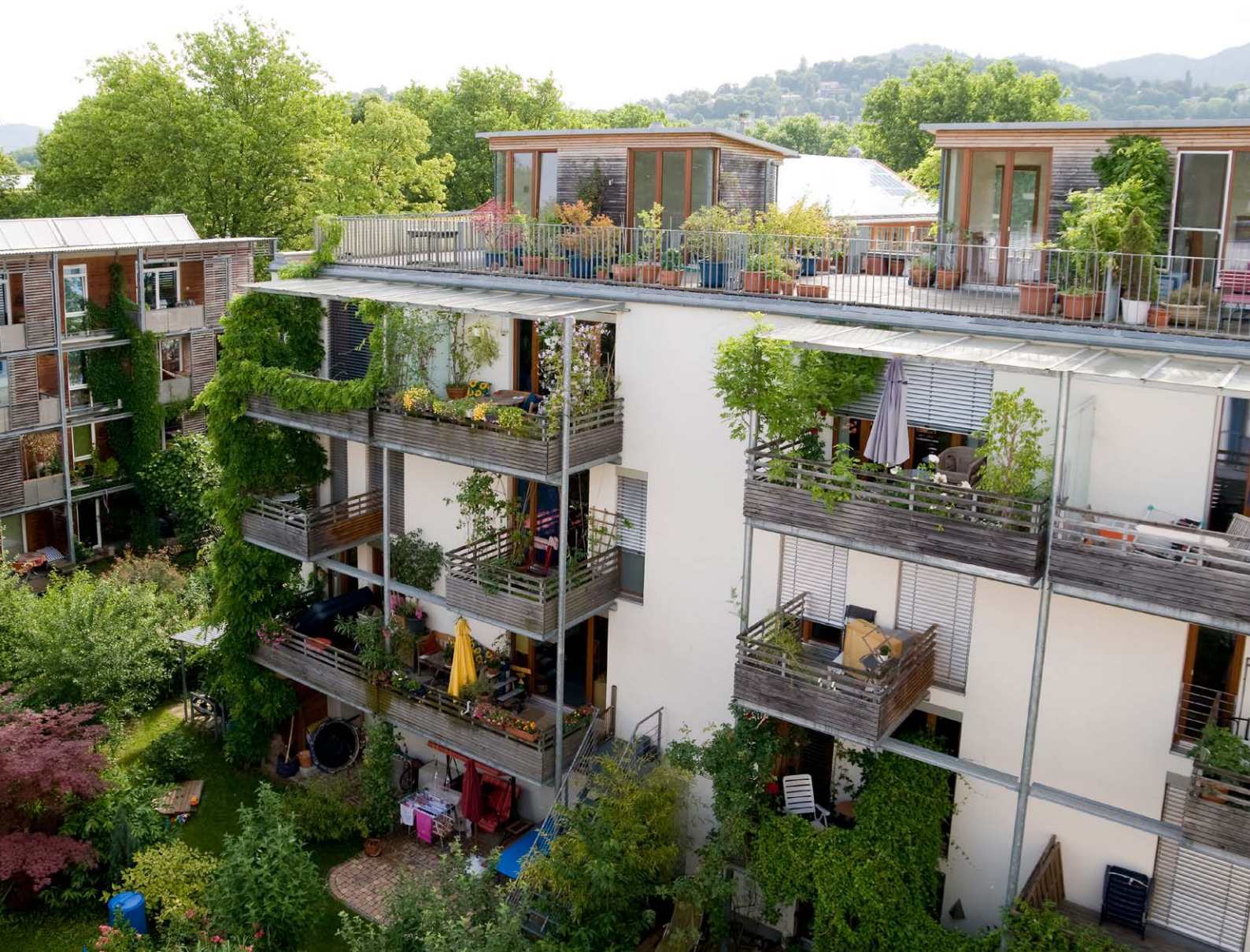
Gardens on the roofs in Vauban
