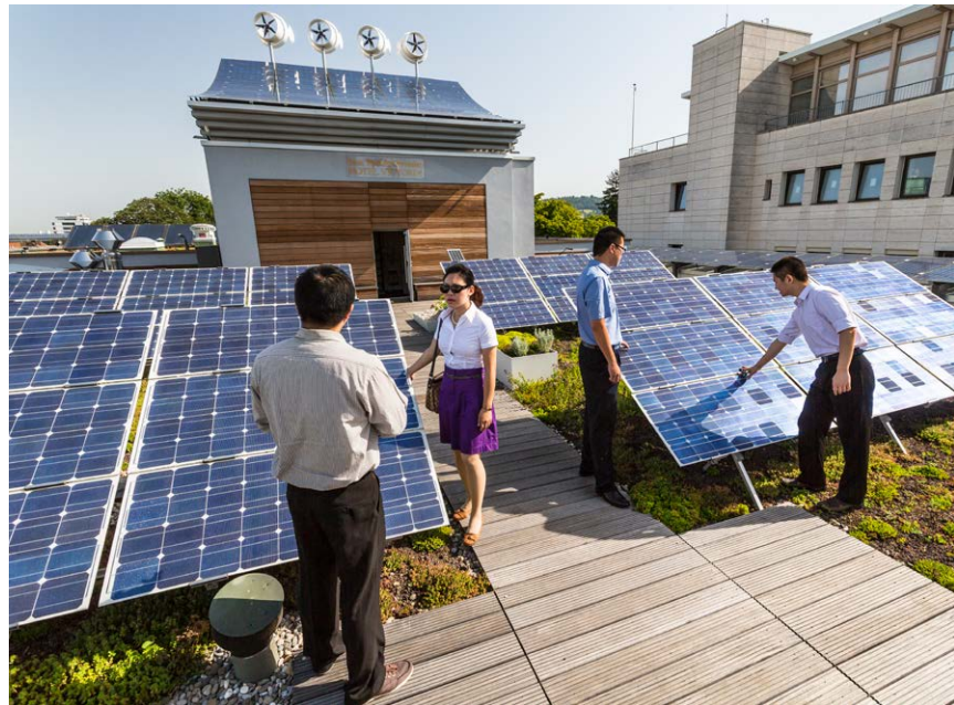
Viewing of a photovoltaic system in the city center
