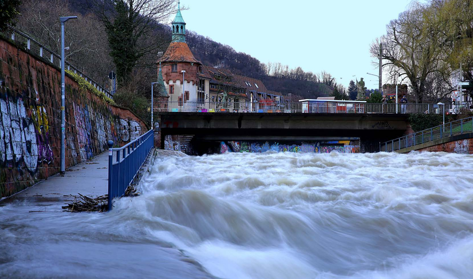
Flood at the Schwabentor Bridge
