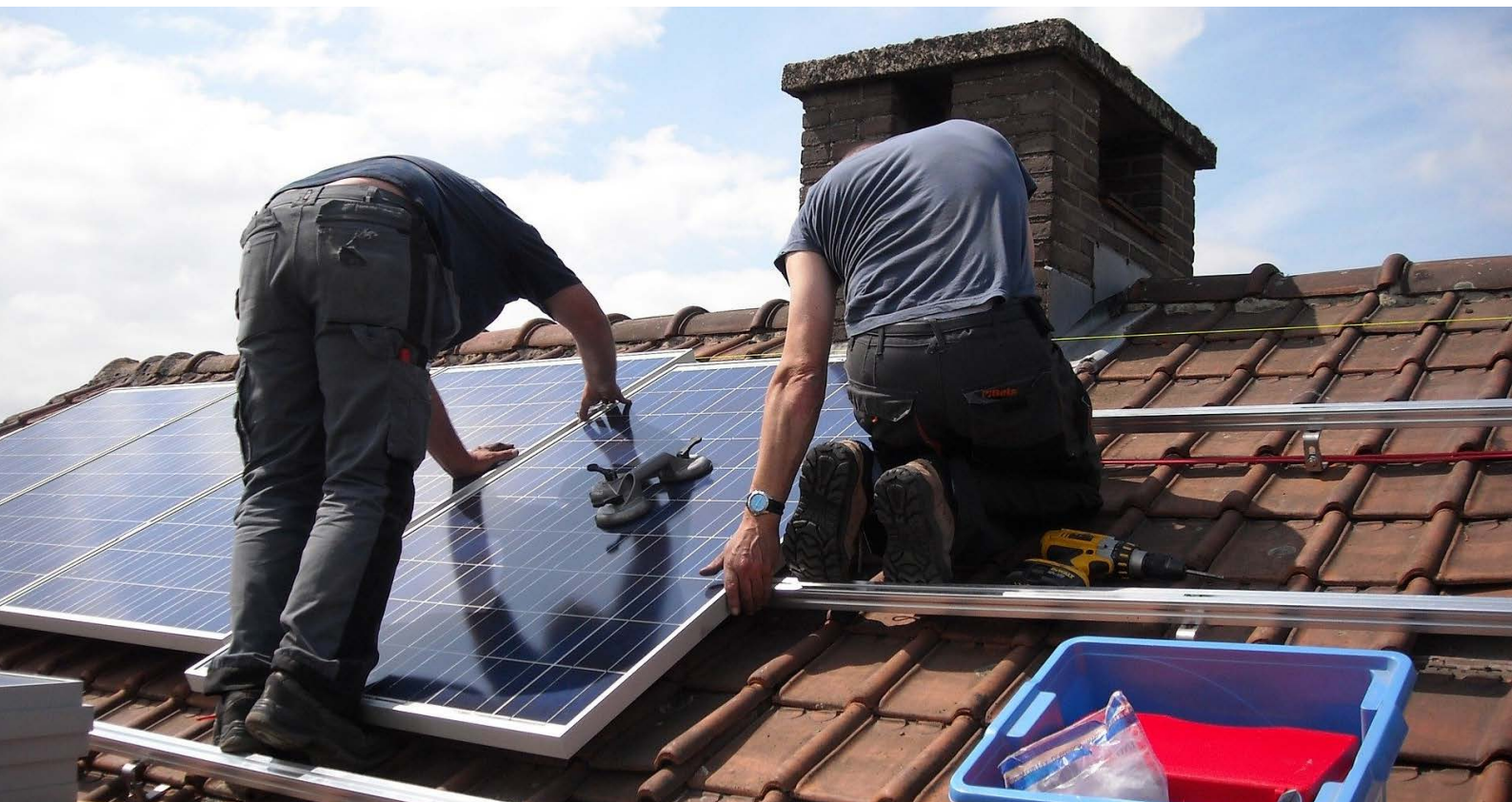
Installation of a photovoltaic system
