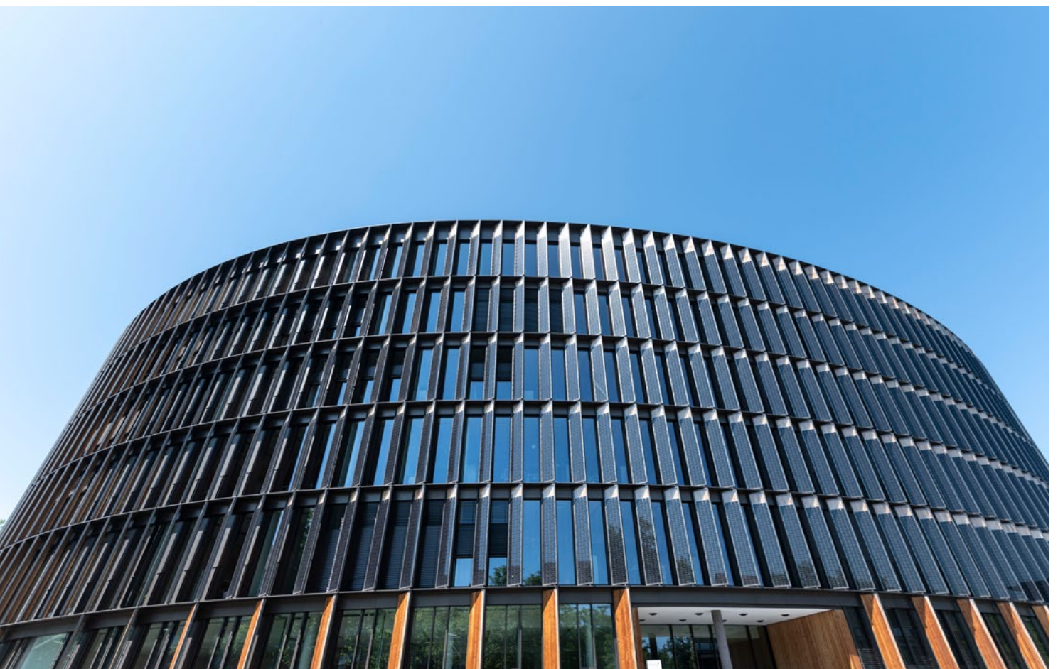
Photo 16: The facade of the town hall in Stühlinger covered with photovoltaics. © Stadt Freiburg, Amt für Bürgerservice
